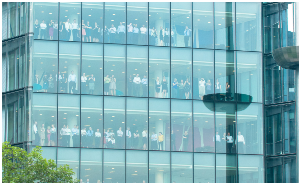
Offices in London Bridge
