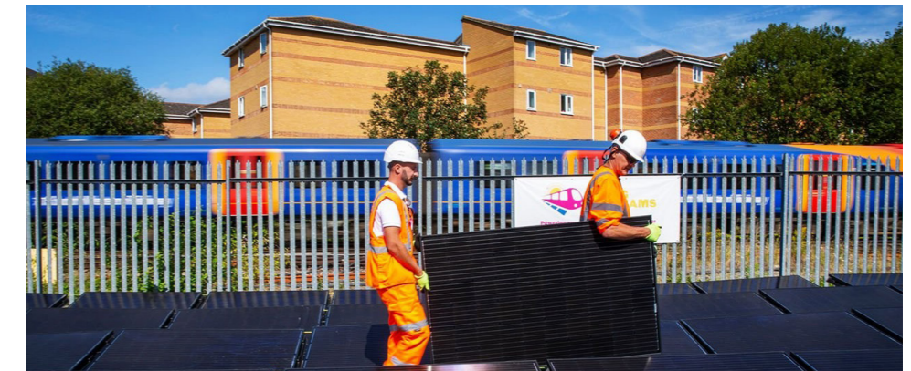
Installation of Solar Panels by Network Rail
